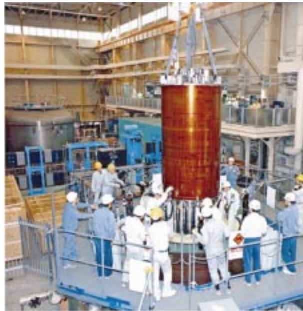
Figure 6. Installation of the CS insert coil into the inner bore of the CS model coil.
