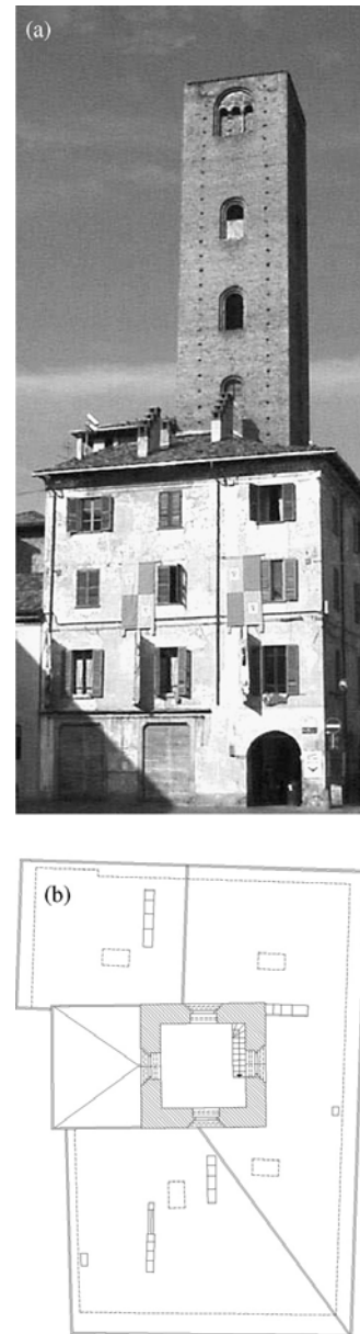
Fig. 1. The elevation view of the tower (a). The plan of the tower and of the surrounding building (b).
