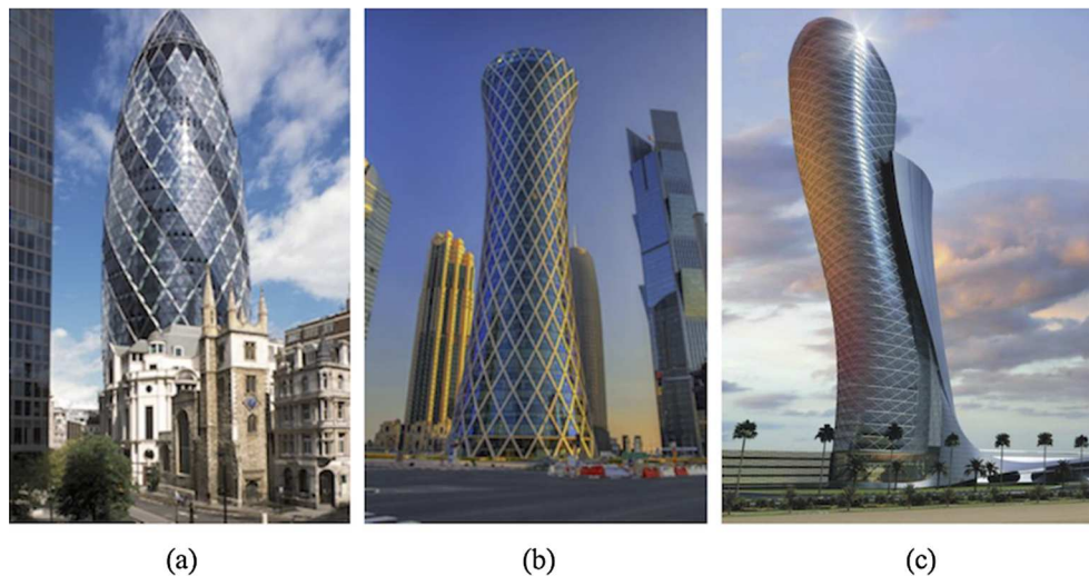
Fig. 1. Examples of diagrid structural systems: (a) Swiss Re Tower, London (from http://larryspeck.com ); (b) Tornado Tower, Doha (from http://www.asergeev.com ); (c) Capital Gate, Abu Dhabi (from https://www.rmjm.com ).
