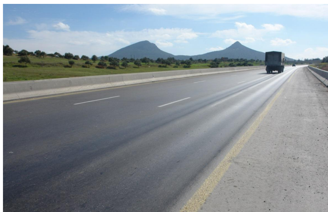
Fig. 1. Presence of ruts on pavement surface due to deformation in the top bound layers (image by Ezio Santagata)
